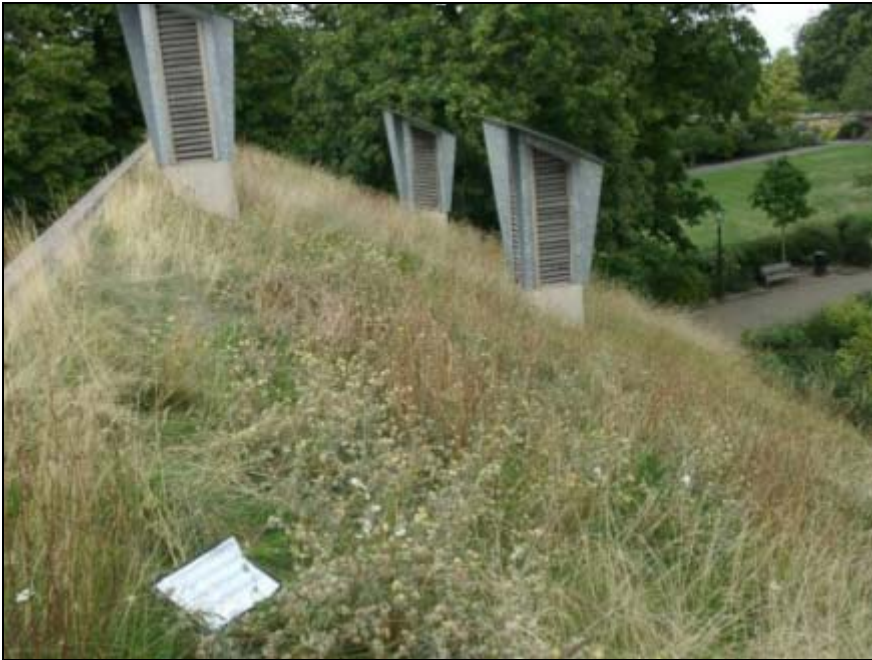
Figure 2: The north-facing section of the roof on the CUE Building, Horniman Museum (photo by B. Nicholson).
