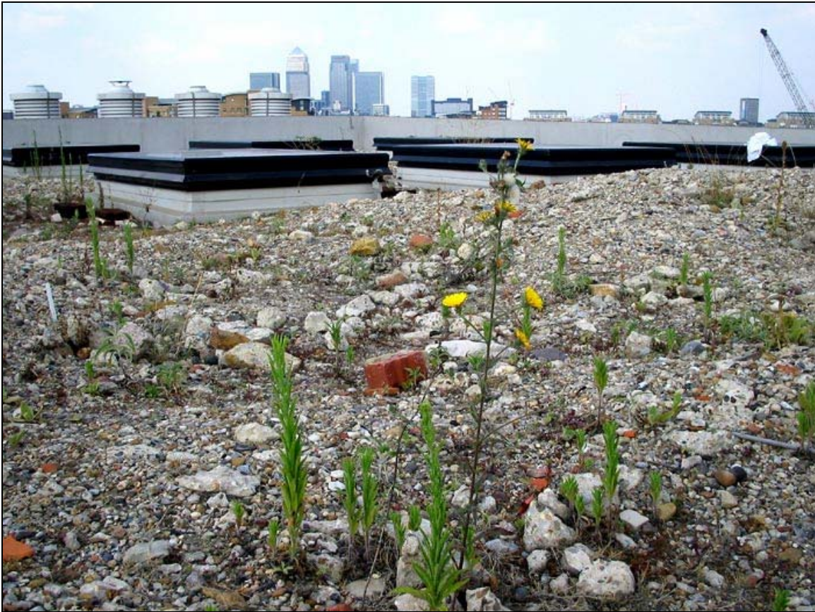
Figure 2: Laban Dance Centre (brown/biodiverse) roof.
