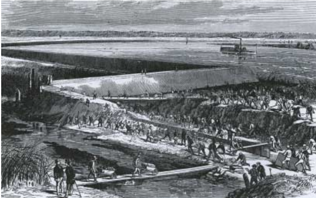
Figure 7: Reclamation of Lower Hackensack Meadows (1), 1867 Photo Credit: Frank Leslie's Illustrated Newspaper , November 16, 1867.
